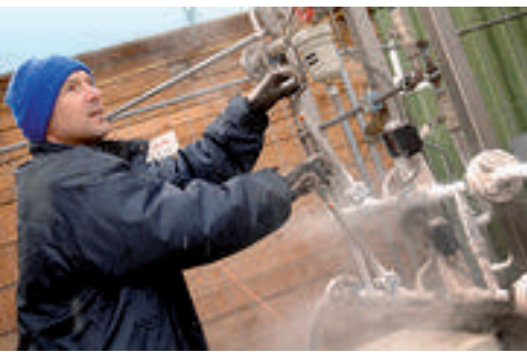
Setting up a cement cooling plant
