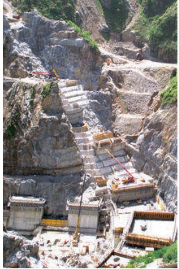
Large construction site at Tsankov Kamak Hydro, Bulgaria
