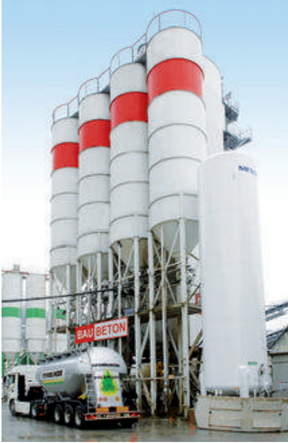
Cooling cement near Innsbruck, Austria
