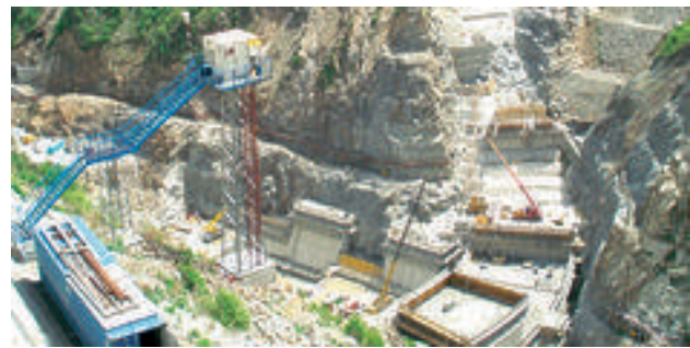
Cooling concrete on a large scale
