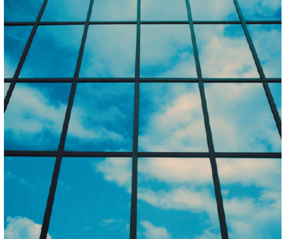
Insulating glass windows filled with noble gases ensure high thermal and sound insulation
