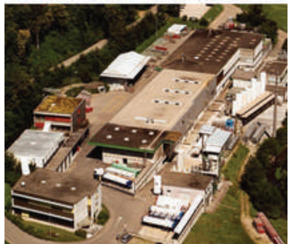
Specialty gas plant Messer Schweiz AG in Switzerland
