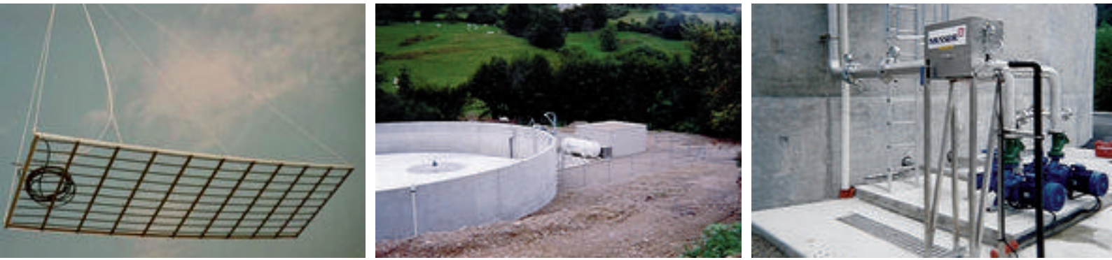
Fig. 6: Neutralization components used by Messer: Aeration hoses (left), Batch tank constructed by customer (center), Liquid feed (right)
