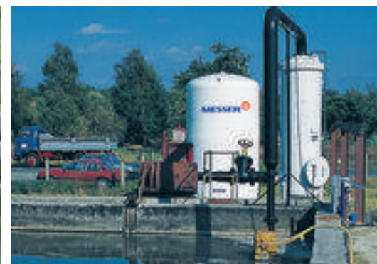
Fig. 1: Pure oxygen input technique developed by Messer: Gassing hose (left), Injector (center), Oxidator (right)
