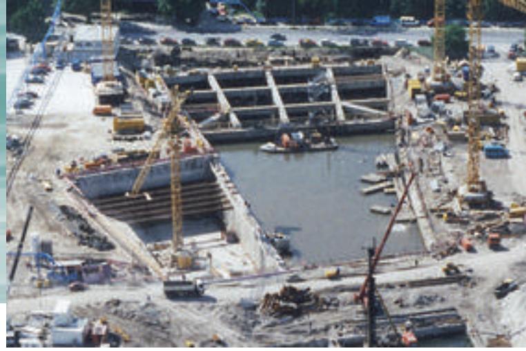
Pre-neutralisation in the underwater concrete basin combined with an in-line neutralisation plant
