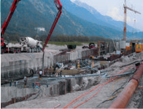
In-line neutralisation at a construction site in Tyrol
