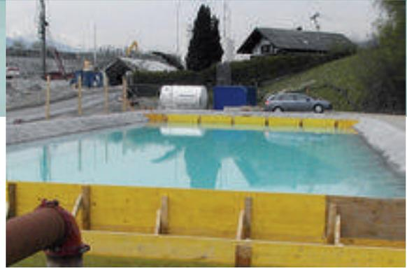
CO<sub>2</sub> storage reservoir of a construction site neutralisation plant
